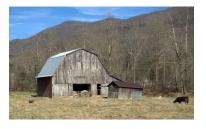
never adapted to hang burley tobacco. The hay loft and roof are uncommon local examples of a structure with no interior posts, using free-standing shallow roof trusses allowing for a larger, open loft. The rail-mounted hay fork and pulley system remain, but became obsolete when baled hay replaced loose-stacked hay.
