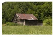
lock sawn lumber. The pattern of lattice around the loft area and gable end is an unusual design. Another hold-over of the earlier type barn includes the use of round pole rafters, many of which are chestnut with the bark remaining in place, a feature of a lost natural history. As typical, the barn was later adapted for hanging burley tobacco. This farmstead also features a very unique and creative early 20<sup>th</sup> century house.
