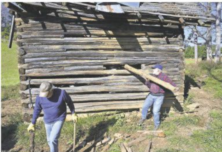
Taylor Barnhill pulls a large log out of the Jarvis-Ray Barn during its deconstruction. COURTESY EVAN PHILLIPS
