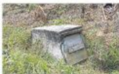
This spring box represented modern plumbing at Claude Wild's farm.
