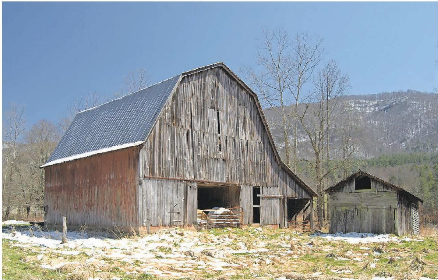
This true gambrel roof barn built Delbert Shelton in the 1950s is unique among the barns of Madison County.
