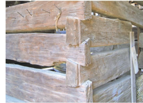
The mortise and tenon joinery inside the barn dates back to the late 1800s.
