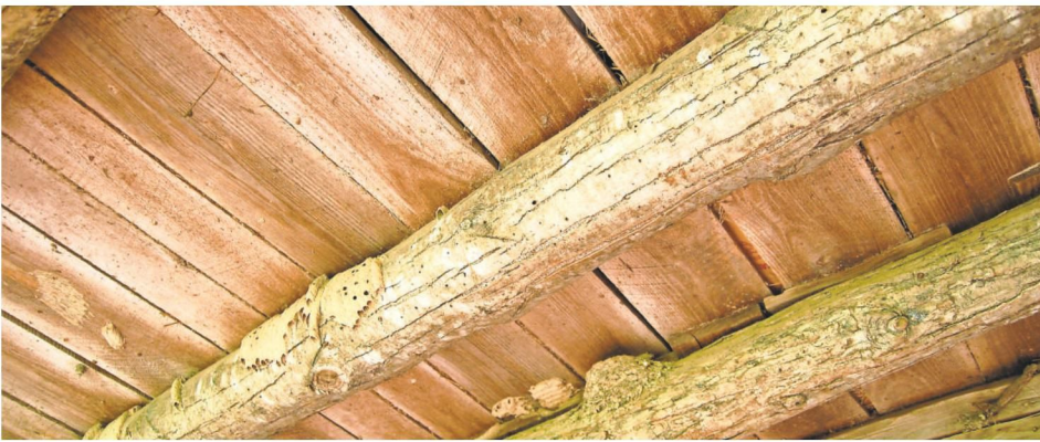
A barn on the Wyatt homeplace features chestnut log floor joists.
