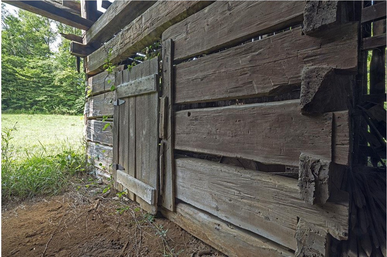
The classic Wallins log crib animal stall with large hewn logs and half-dovetail notching.
