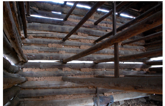
24" tier pole spacing, unique to flue-cured tobacco
