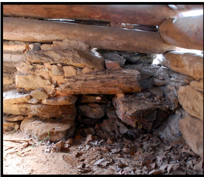
Surviving rock furnace opening in rock foundation
