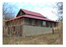
tween the logs, or that it was ever used to heat cure tobacco. The shed roof additions on all four sides appear to have been built early in the existence of the central log section. There are no log crib animal stalls, except for the one large crib on the ground level. The second floor has been used as a hay loft, and likely a grain threshing floor, over its lifetime.
