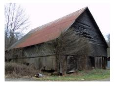
with a wooden floor. The barn has good examples of mortise and tenon joinery and, as was typical, the vertical posts are sawn, while long plates, sills, and some long beams are hewn. This is a common bank barn, the bank supported by a massive rock wall. Tier poles appear to have been added to hang Bull Face or Rockwood chewing tobacco. The original wood shingle roof was replaced with metal roofing around 1946.
