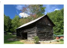
notch with several V-notch corners. The rafters are round poles, an uncommon feature for this period, especially with the tightly spaced roof sheathing, originally installed for tarpaper roofing. The farmstead is at an elevation of over 3300 feet, in a steep valley in a remote corner of the county.
