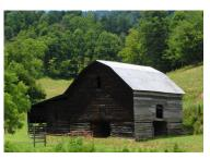
coincided with the availability of a new roofing material, metal sheet roofing, which began to replace the standard roofing material — split oak wood shingles, after WWI. The barn is also a quasibank barn with a high bank behind connected by a log bridge to the road above. The log cribs are set upon large square-hewn wood sills on field stone piers. Two additions were added at different times on the south side, as additional hanging sheds were needed for air-curing burley tobacco.
