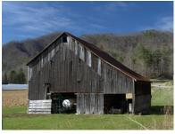
ber framing is with mortise and tenon joinery, and one stall door survives with its very rare wooden hinge. Unlike most barns of this period, there is no lattice work. The hay fork is still in place, which is uncommon, as are the 19<sup>th</sup> century style hay racks with angled split palings. The Shelton family has been the influential family in the Shelton Laurel valley since the early settlement period.
