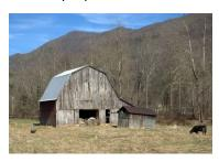
roof are uncommon local examples of a structure with no interior posts, using free-standing shallow roof trusses allowing for a larger, open loft. The rail-mounted hay fork and pulley system remain, but became obsolete when baled hay replaced loose-stacked hay.
